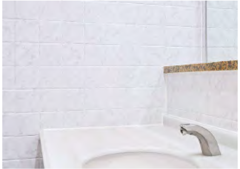
Restroom refurbishment / ST-024TIL
